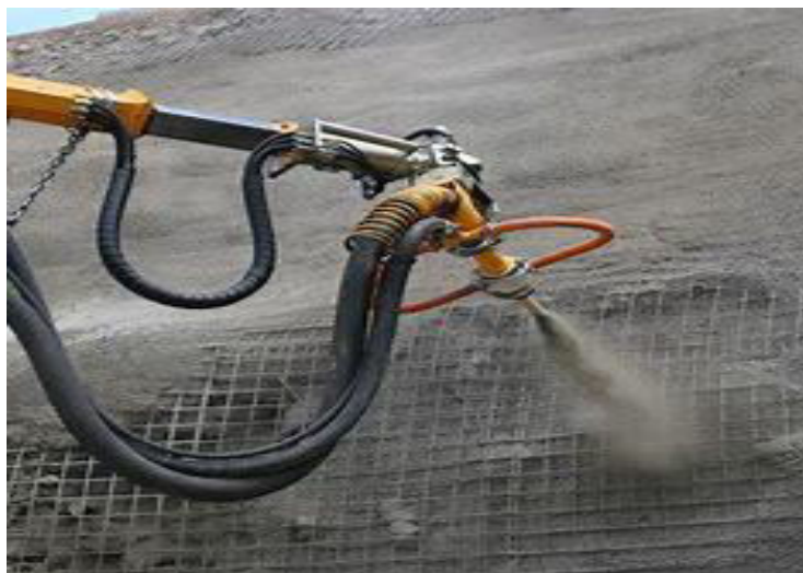
Fig No. 4. Shotcrete
